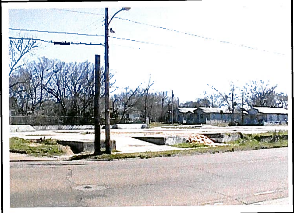
1400 Block of N. Mill Street
